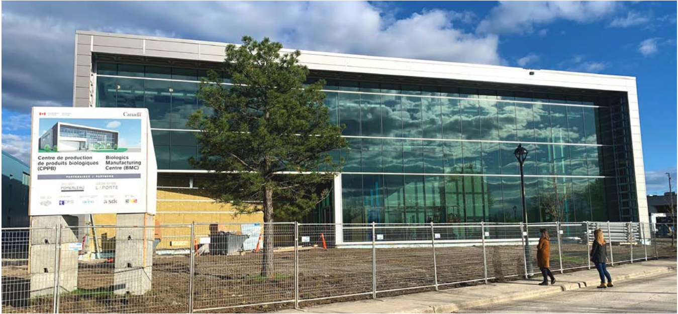
The Biologics Manufacturing Centre at Royalmount, under construction.
