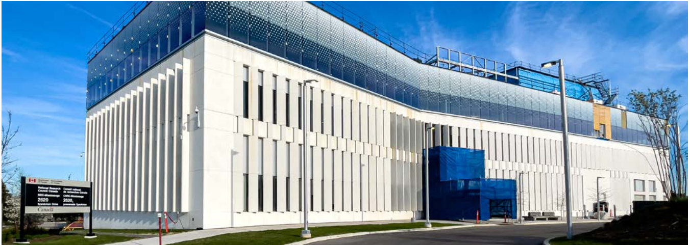
The National Research Council of Canada's new advanced materials research facility in Mississauga.
